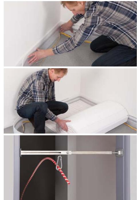
Efficient unwinding of the Pe-Xcellent and the aluminium composite hook-and-loop piping are made possible with the intelligent pipe unwinding aid.
